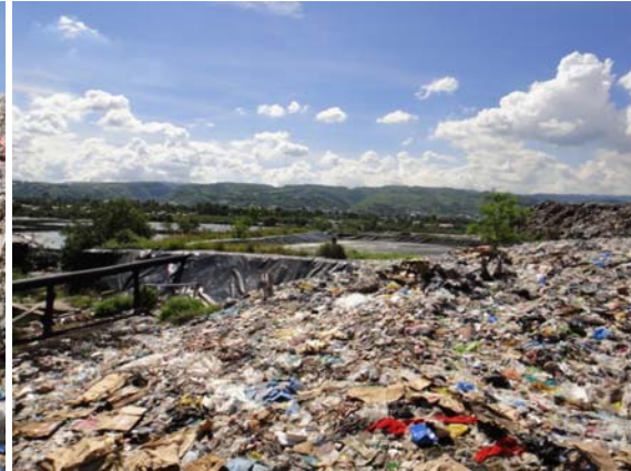
Figure 4: Abandoned Leachate Treatment Pond in the Landfill Site. Photo: Premakumara, 2010
